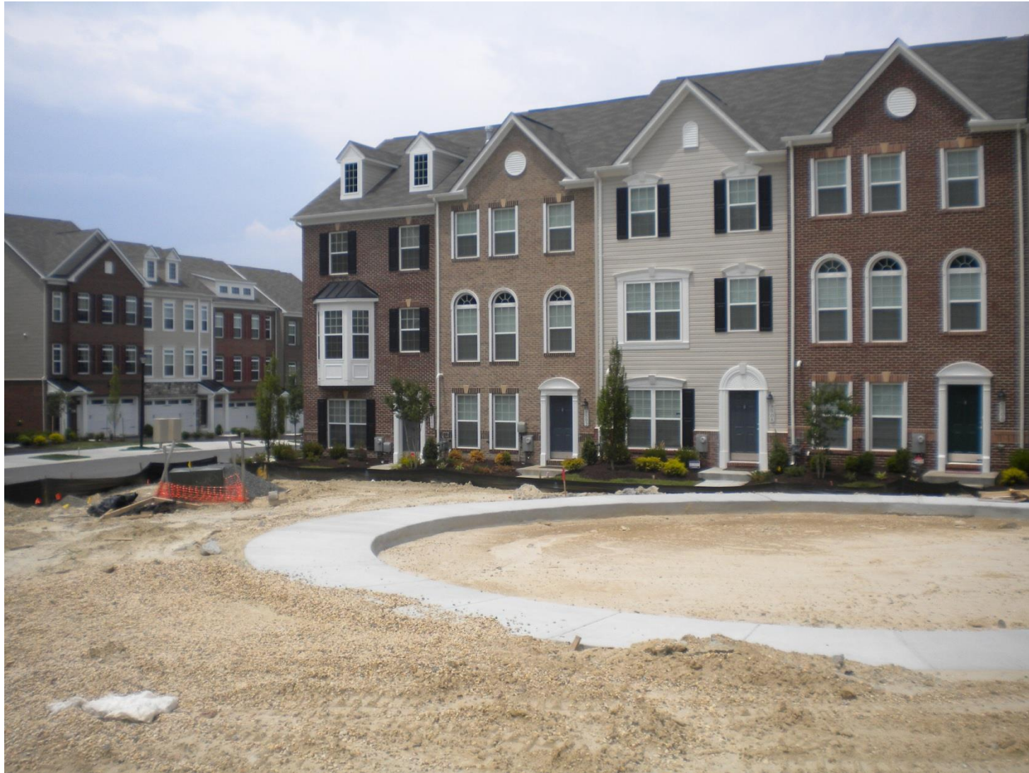
Phase I South of Fernwood Drive under Construction with a Play Area in the Foreground
