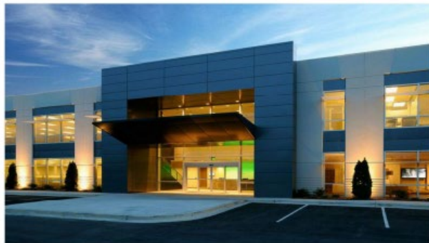
EXAMPLE OF MASSING AND MATERIALS- HORIZONTAL REVEALS
