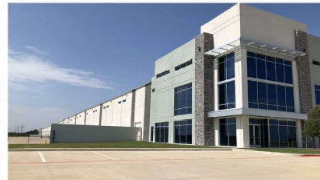
EXAMPLE OF MASSING AND MATERIALS- ALUMINUM SUNSHADES
