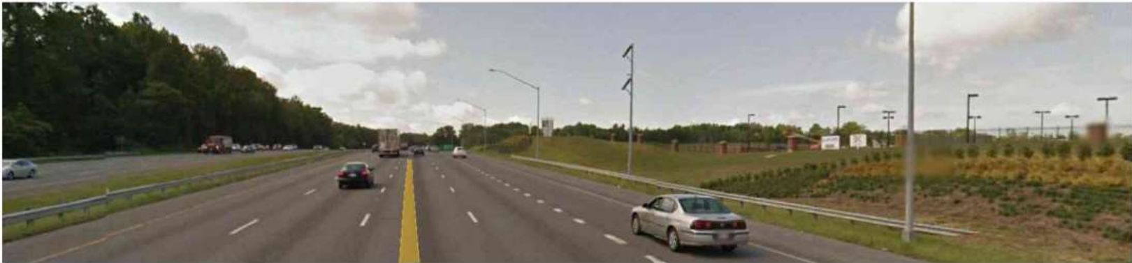
Southbound I-495 @ Viewing Distance of 955' EXISTING SIGN
