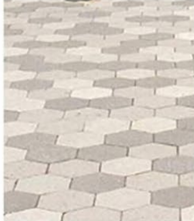
Front Plaza: Multisided Prest Brick by Hanover
