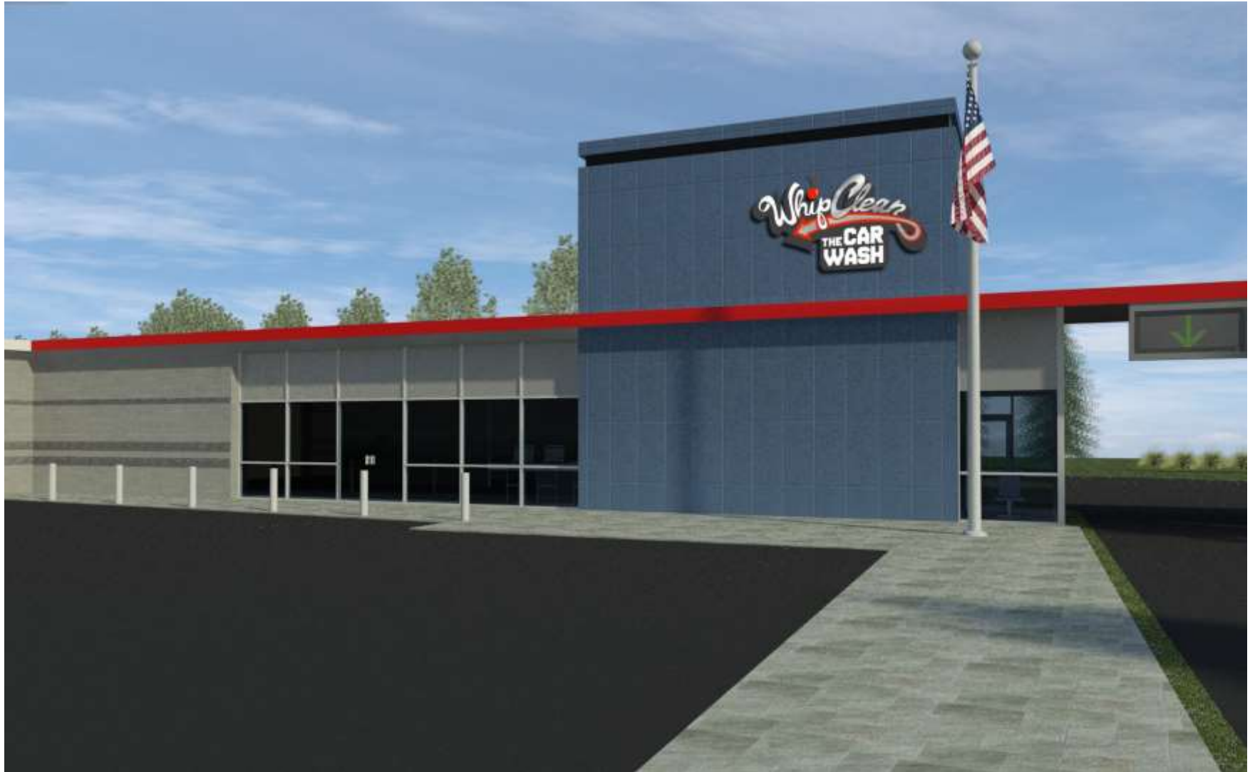
Area of the Office Entrance
