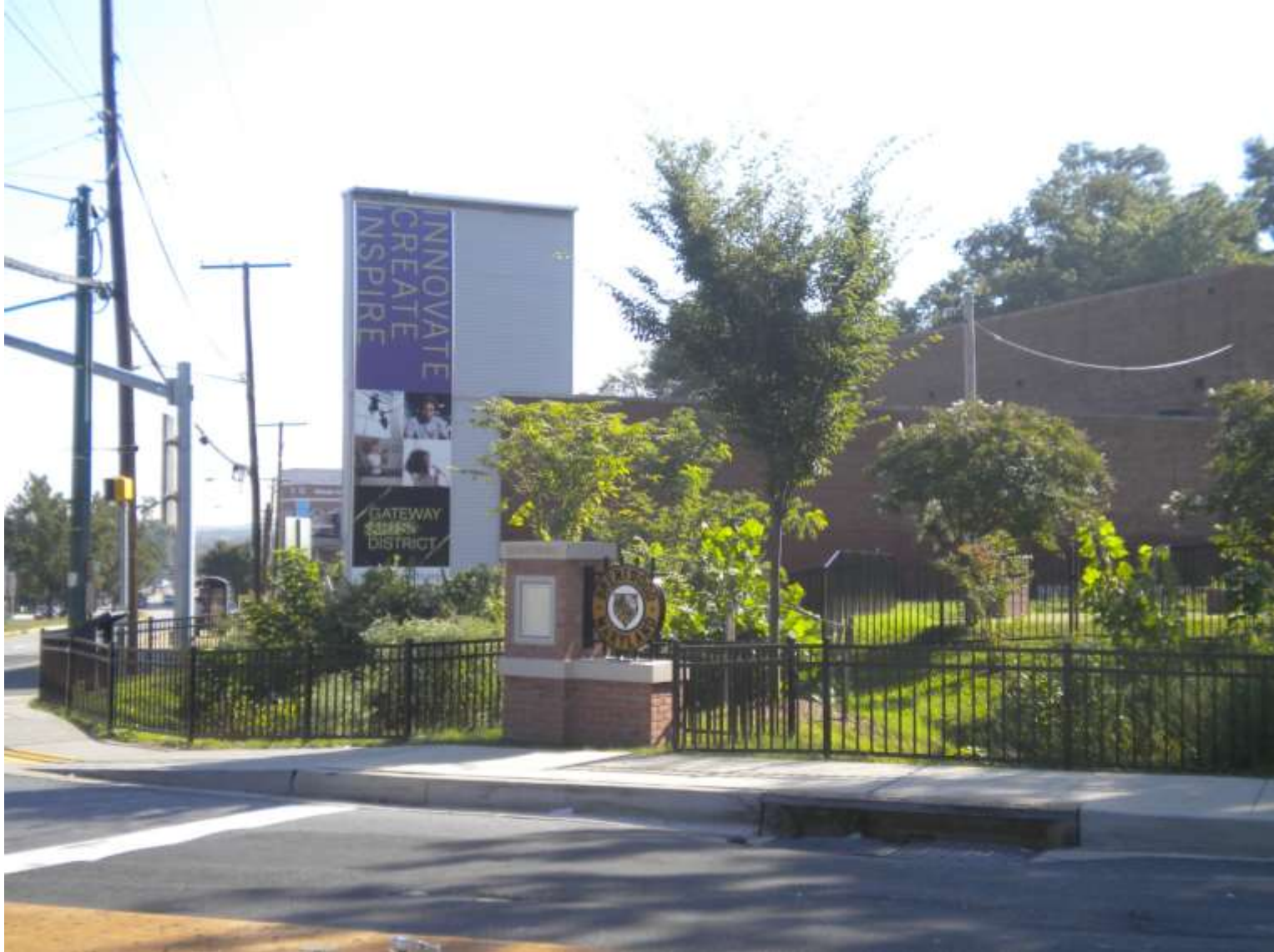
Existing Stormwater Park at the Intersection of 38 th and Rhode Island
