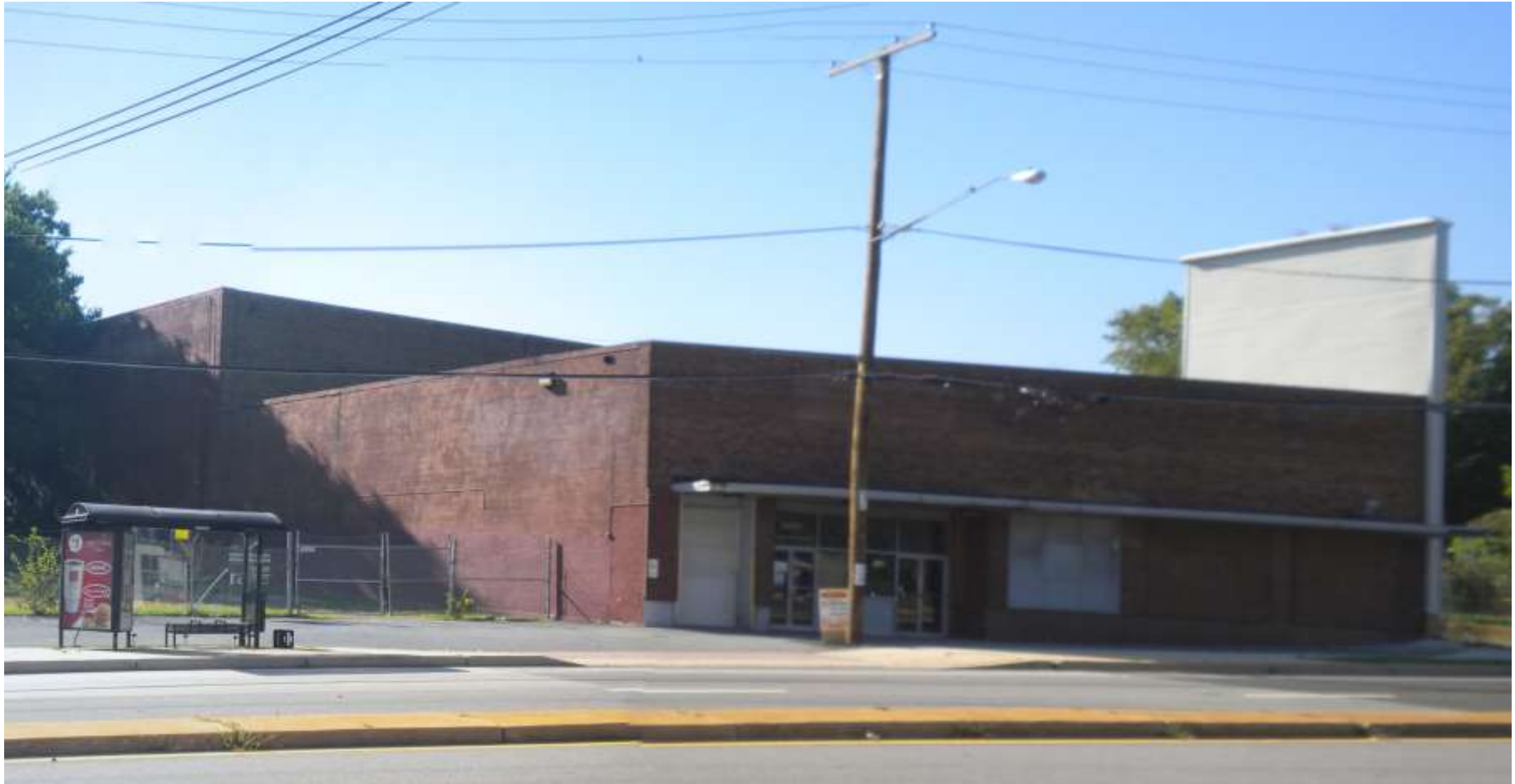
Existing Warehouse Building to be Razed
