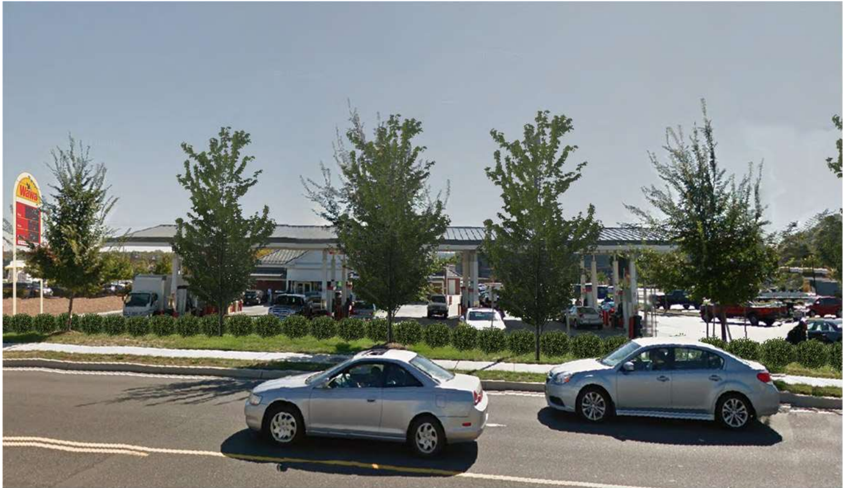
Allentown Andrews Gateway Center Exhibit "B". View from Allentown Road into site
