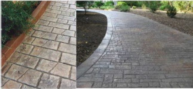
CROSSWALK-STAMPED CONCRETE EARTH-TONE COLOR/PATTERN TO BE DETERMINED
