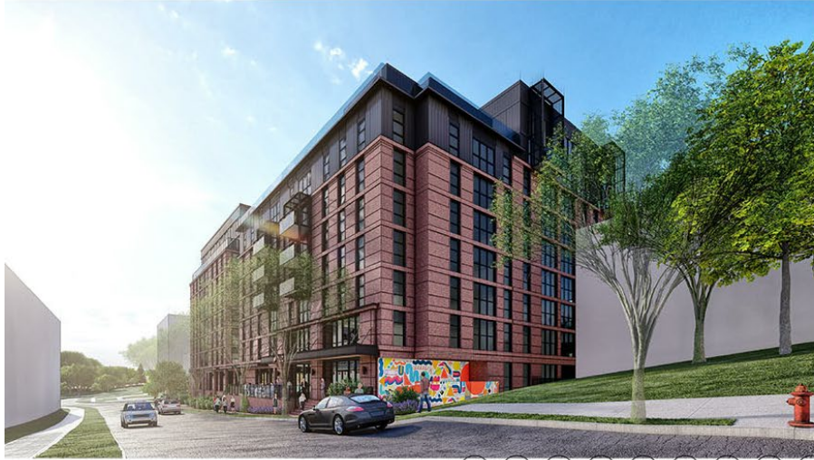
VIEW LOOKING NORTHWEST FROM KNOX ROAD
