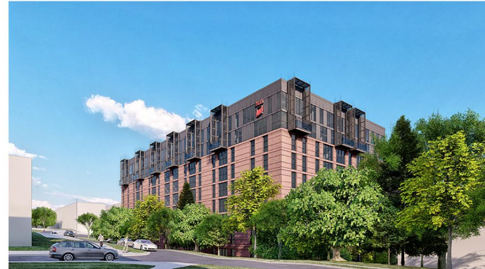
VIEW LOOKING SOUTHEAST FROM LEHIGH ROAD
