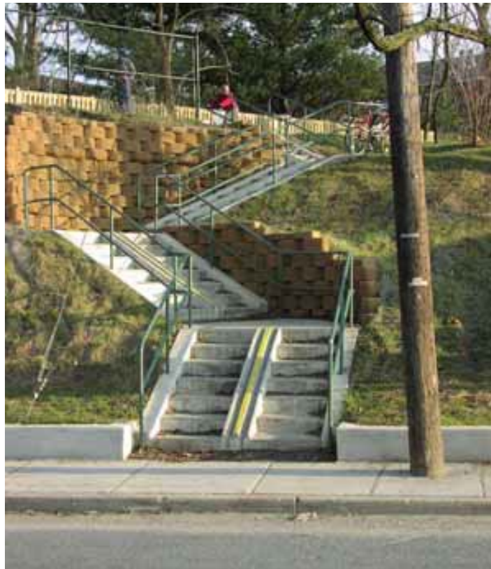
This photo gives an example of a bicycle trough, which enables bicyclists to easily walk their bicycle up or down a set of stairs by providing an area where the wheels of the bicycle can be placed adjacent to the stairway.
